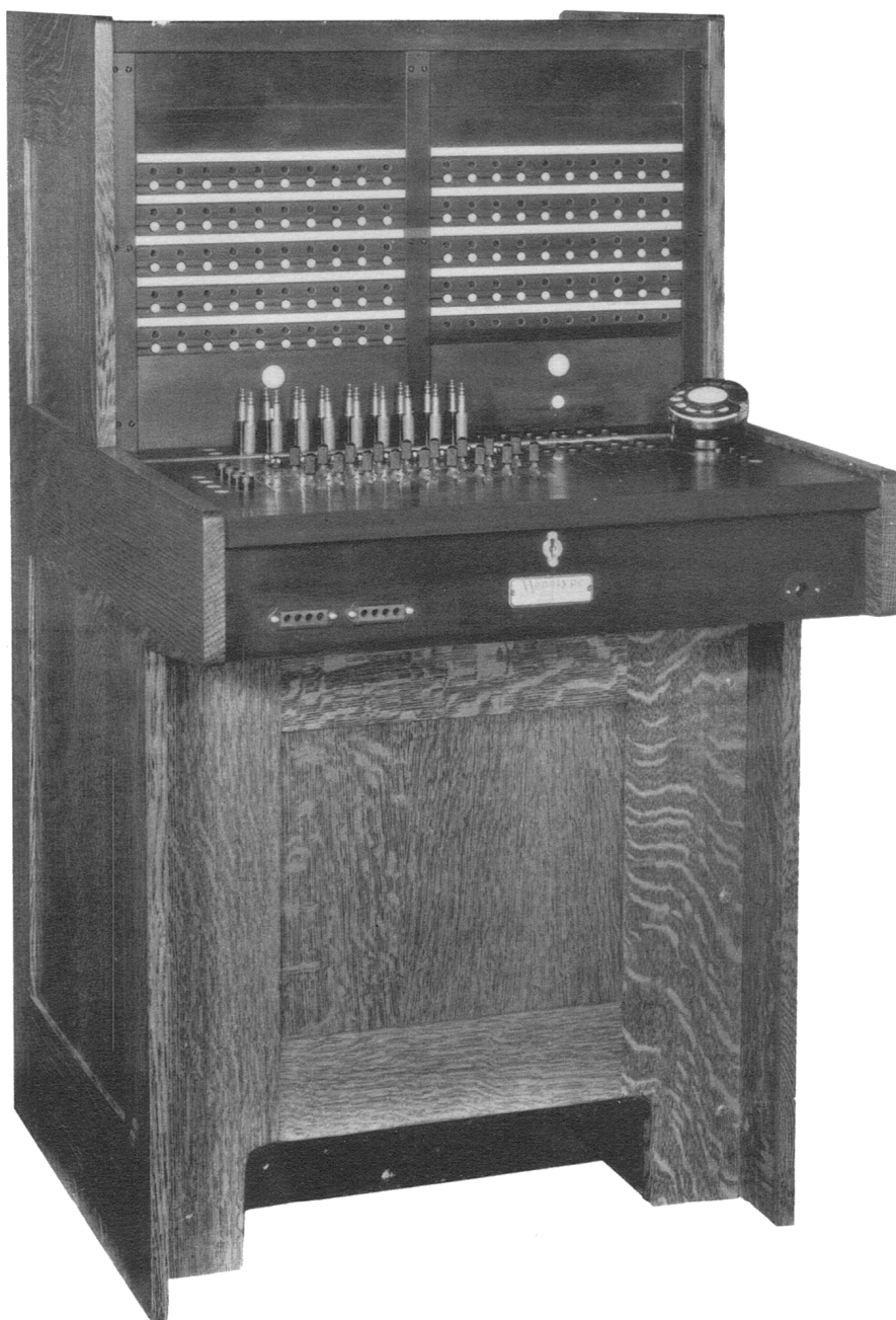
100-LINE MONOTYPE P.B.X. 80 LINES EQUIPPED. 10 TRUNKS EQUIPPED. 10 PATCHING JACKS. 9 FEATURE CORD CIRCUITS ARRANGED FOR AUTOMATIC OPERATION
